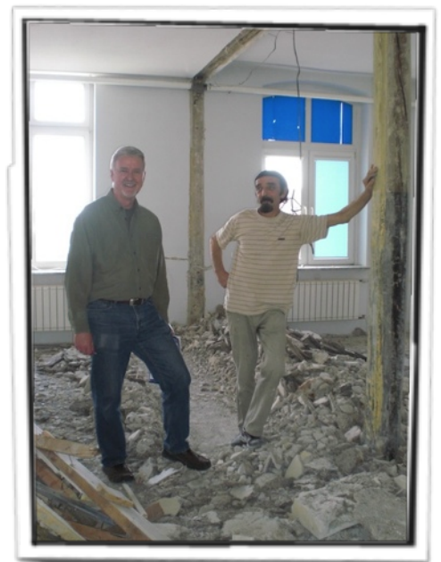
Joseph checking on the progress of demolition
